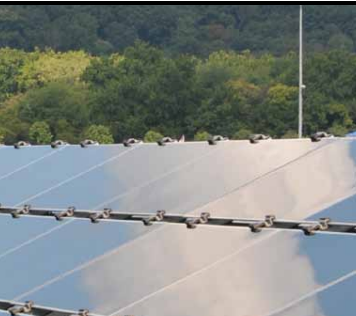
Generating Clean Horizons, a 16.1-MW project at Mount St. Mary's University in Emmitsburg, Md., received one of PV America East's 2013 PV Projects of Distinction Awards. Photo courtesy of Mount St. Mary's University.
